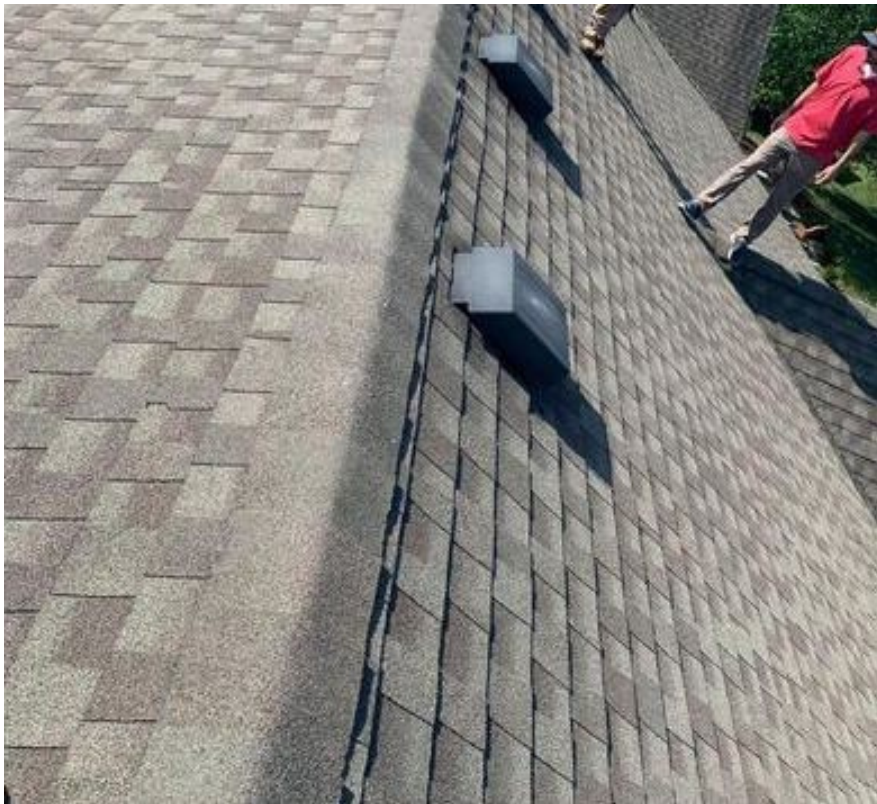
Component(s): Box Vent, Shingles Overview
