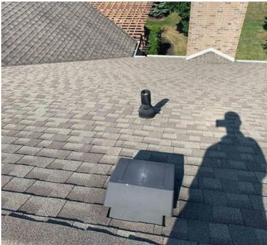
Component(s): Shingles Overview, Pipe Vent, Box Vent
