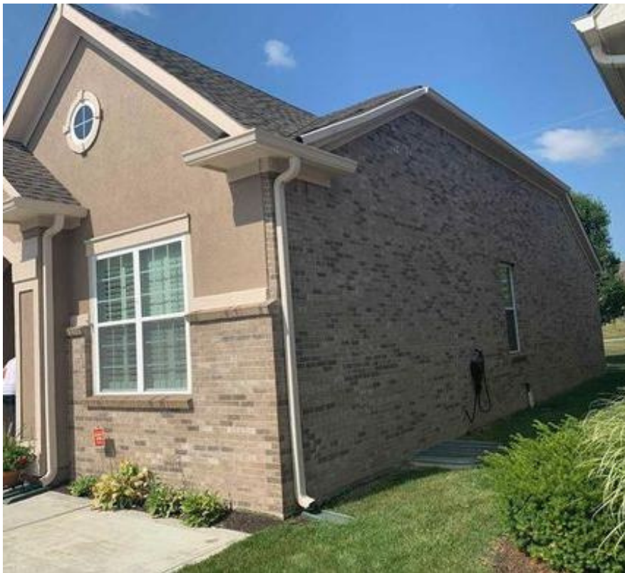
Component(s): Downspout, Fascia, Siding
