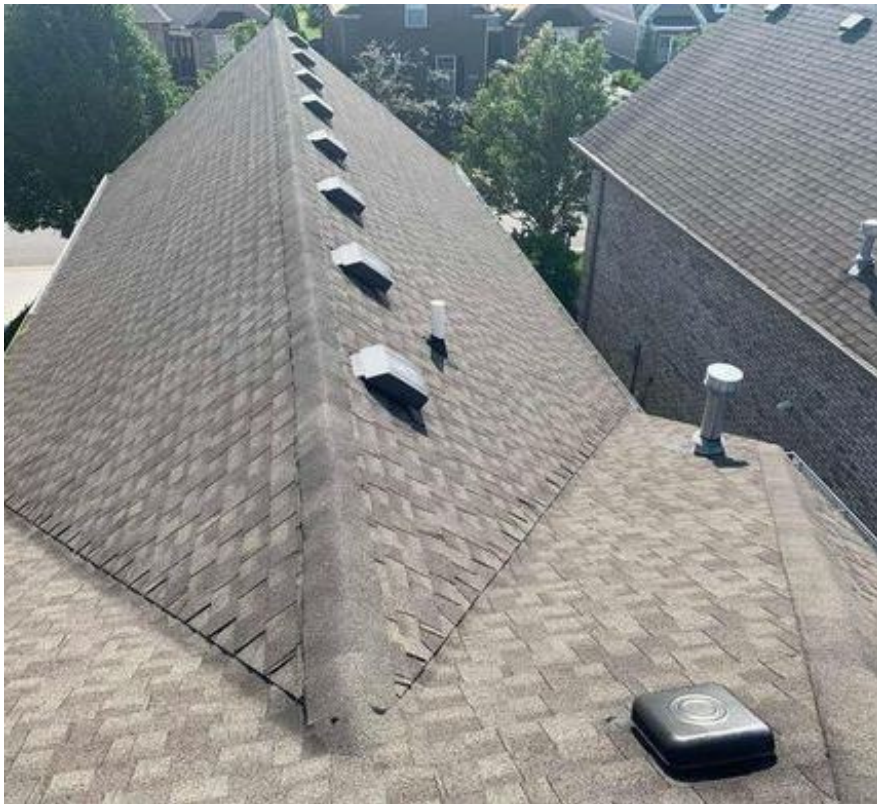
Component(s): Shingles Overview, Box Vent, Hvac Vent, Pipe Vent
