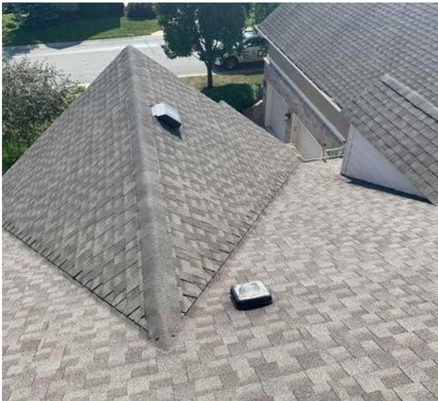
Component(s): Box Vent, Shingles Overview
