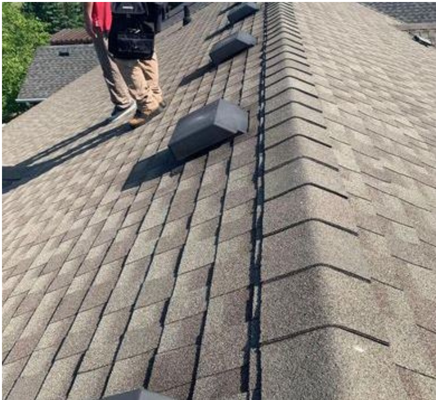
Component(s): Pipe Vent, Box Vent, Shingles Overview
