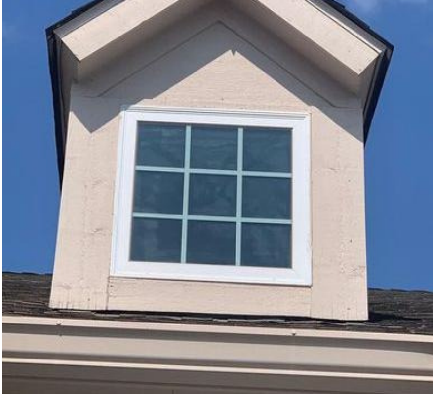
Component(s): Window, Siding, Fascia, Gutters
